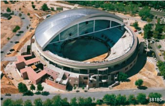
Protection against sun and rain: The roof sections can be gently turned into position, as needed.
